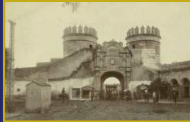
Inner façade of Puerta de Palmas in 1903. The side entrances had not been opened yet, and so the gate was joined to the rest of the wall. We can also see the walled-off upper chapel and the guardhouses by the gate. Javier García Ramos's Collection.
